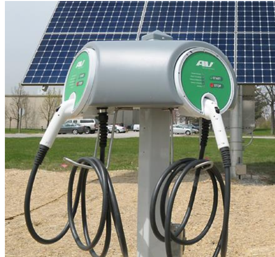
Pedestal-mounted Level 2 EVSE paired with solar and used for workplace charging (Argonne National Laboratory Photo)
