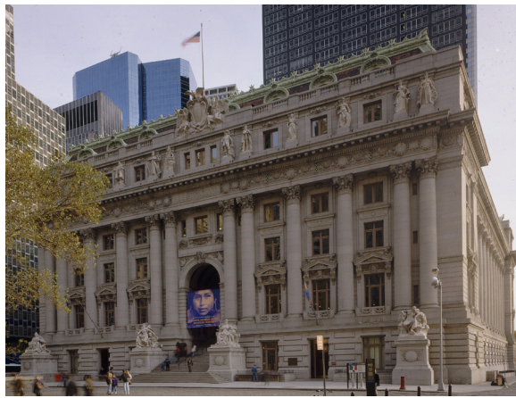
Left: The Hirshhorn Museum and Sculpture Garden is eligible for listing on the National Register for Historic Places and is in the National Mall Historic District. Current projects will improve its resiliency to flooding as well as heat. Right: The National Museum of the American Indian is located in the lower levels of the Alexander Hamilton U.S. Customs House in Lower Manhattan.
